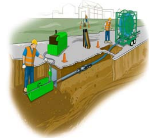
STATIC PIPE BURSTING
